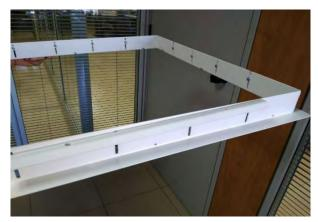
2.- Install the part that goes fixed to the VL-PRO with the rods included in the VL-PRO. These 4 rods need to be cutted at the requiered size of the installation.
