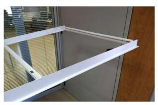
OPTIONAL.- You can add the optional third metal bar, in case you want to make it easier the manipulation of the end of run or of the projector. Adding this piece you can put the ceiling piece in 2 parts. So in case you need to make any maintenance you can make it only removing one part of the ceiling.
